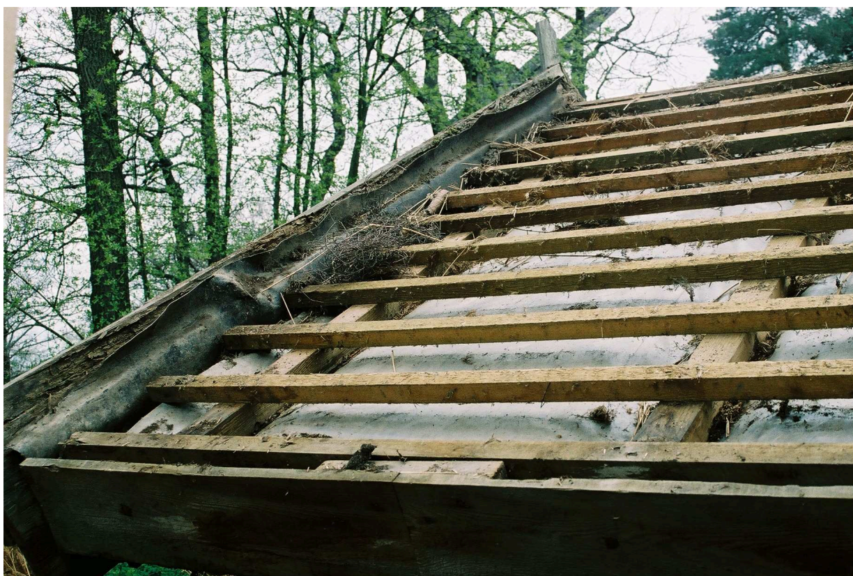
Taket under rivning.
